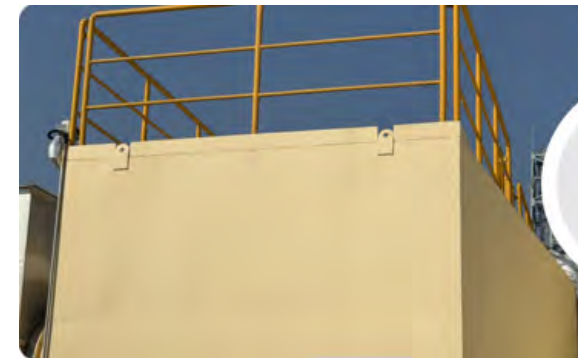
Primary activated carbon
